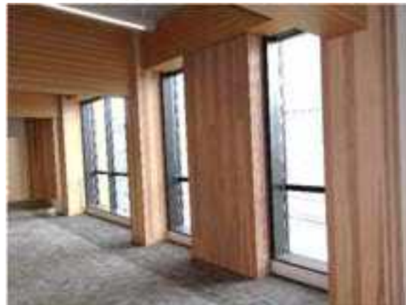
CLT (Cross Laminated Timber) 耐震壁
